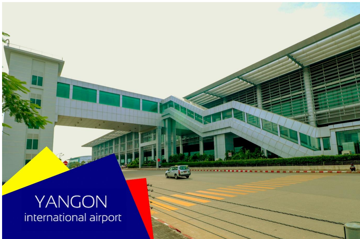
The Link Bridge directly connecting the car park and Terminal 1, Level 4 at Yangon International Airport
