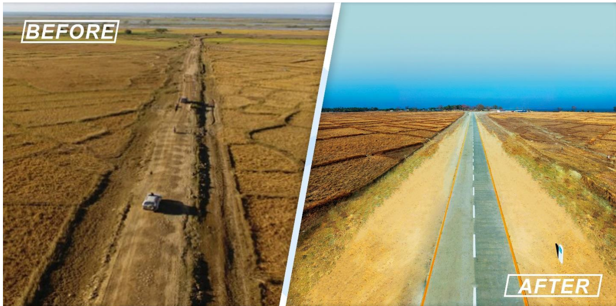
Photo: The before and after picture of the 54 KM all weather concrete road connecting Angumaw to Maungtaw
